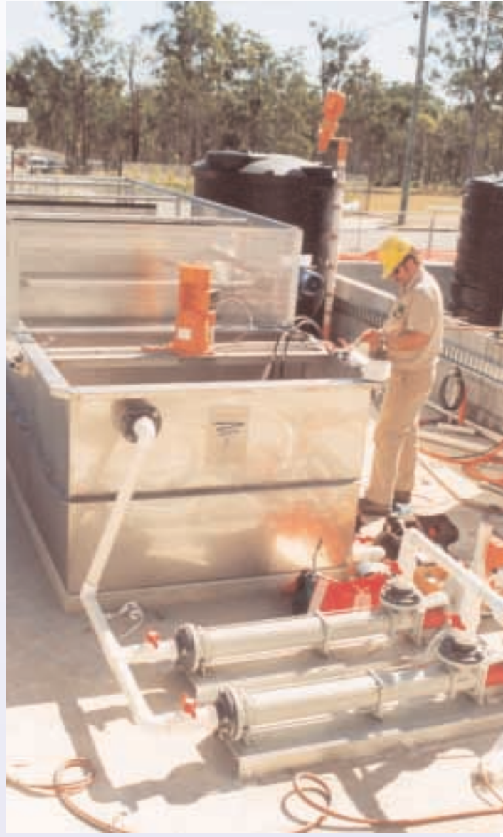
SNAP FRESH WWTP under construction in Queensland
